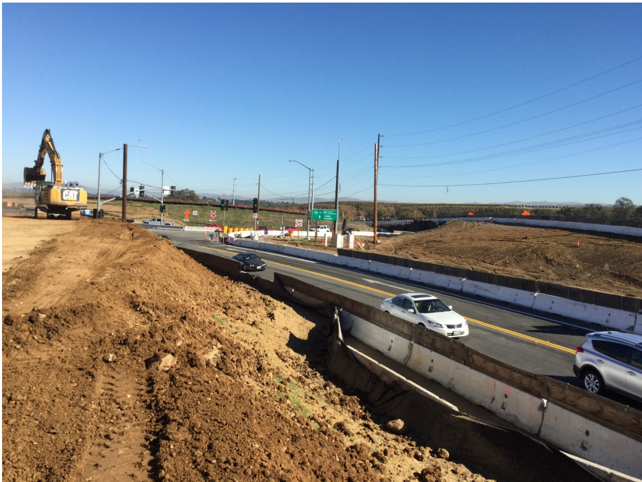
(SR 84 Expressway Widening, courtesy of ACTC)
