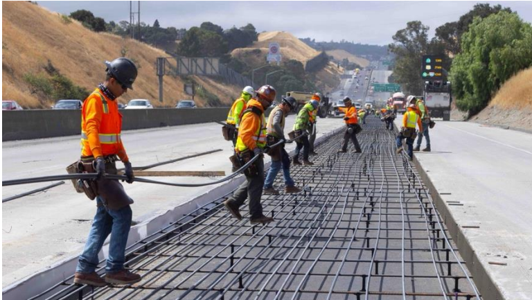
Pavement & Bridge Rehabilitation
