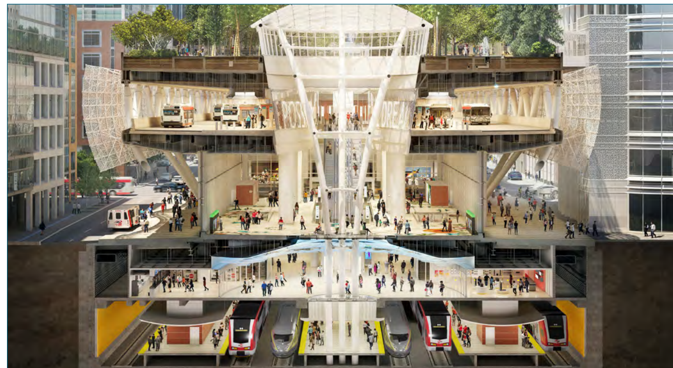
The Salesforce Transit Center includes a two-level trainbox, which will house the future train station mezzanine and the train platform. (Rendering courtesy of TJPA)
