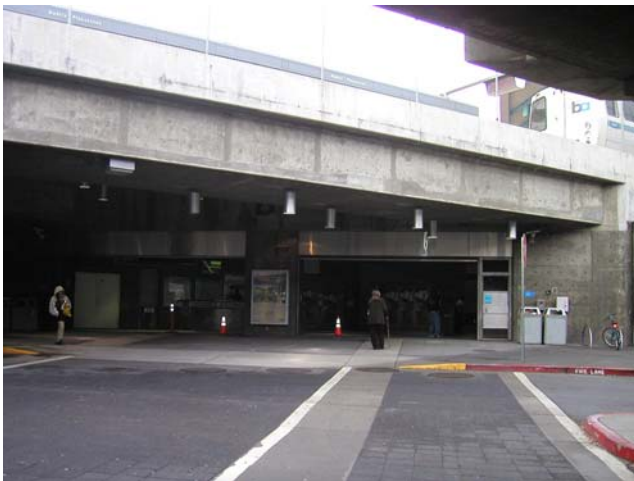
7. BART station entry/exit. Needs wayfinding and directional signs to bus platforms.
