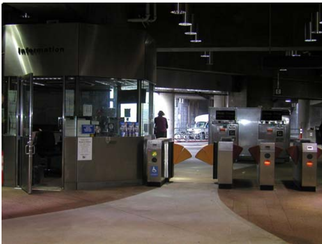
17. Existing BART station agent booth. Create a place for temporary signs and messages.
