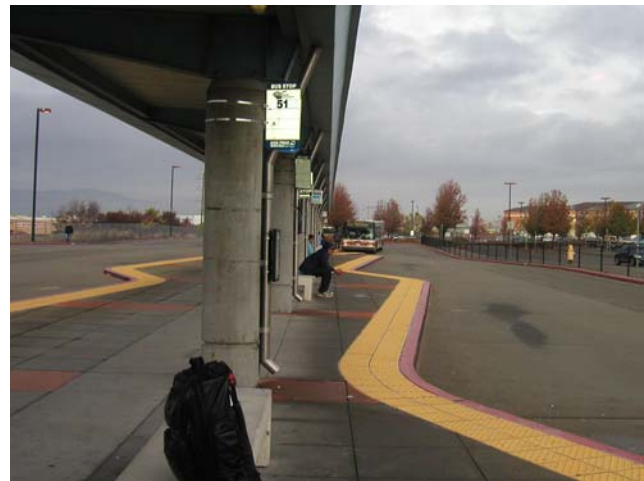
8. Existing bus stop signs are not bold enough.
