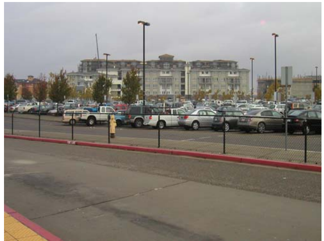
2. Walkway entry from parking lot, lack direction signs to station entrance.
