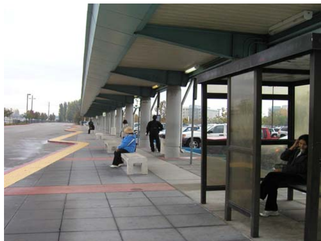
10. Existing bus shelter. Existing bus canopies do not provide adequate shelter from weather and do not provide adequate transit and bus information.
