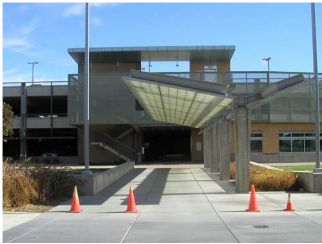
5. View from bus bays to Transit Store and parking structure.
