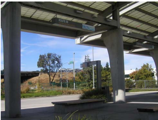
13. Overhead route identification.
