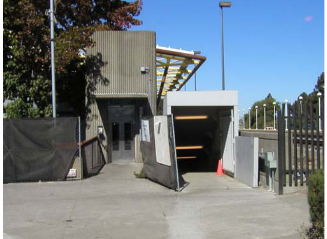
10. Entrance from bus facility to BART/Amtrak lobby. Note lack of wayfinding signage.
