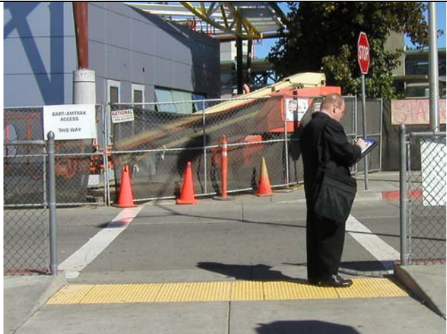
2. Temporary BART/Amtrak entrance during construction
