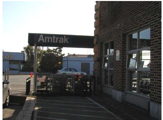
7. Amtrak ticket office just south of Ferry Building. Signage is not highly visible from all directions.
