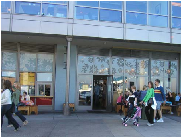
6. Lack of wayfinding signage for arriving ferry passengers.
