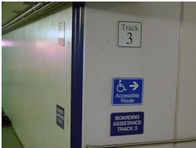
7. Existing: Tunnel access to train boarding platforms.
