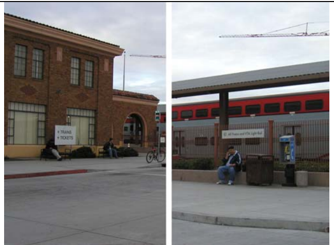
2. Signage at side entrance
