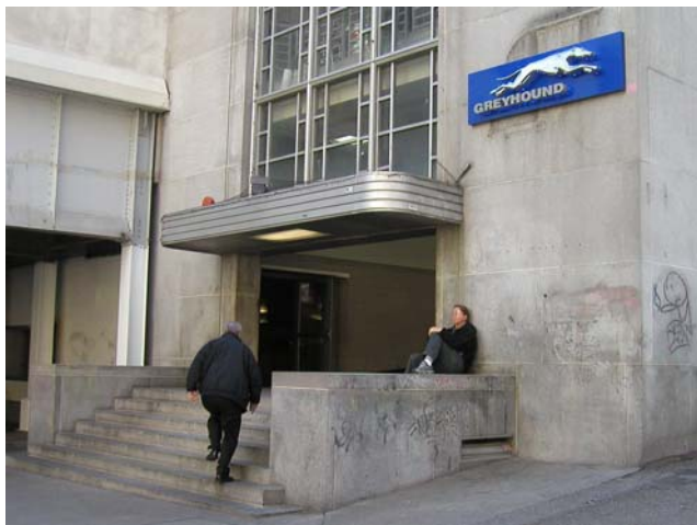
4. Side entrance. Note lack of station name/id.
