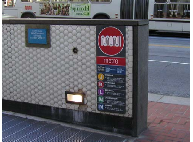
22. Listing of Muni trains on side of entry stair.
