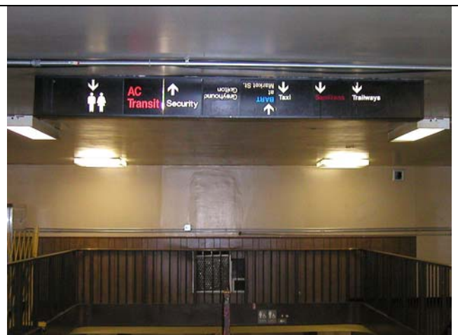
10. Exit sign. Note upside down signs, lack of arrows.
