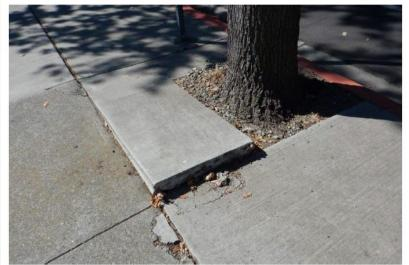
Example of tripping hazards on sidewalk caused by existing trees (Sidewalk to be reconstructed to preserve trees and meet ADA requirements)
