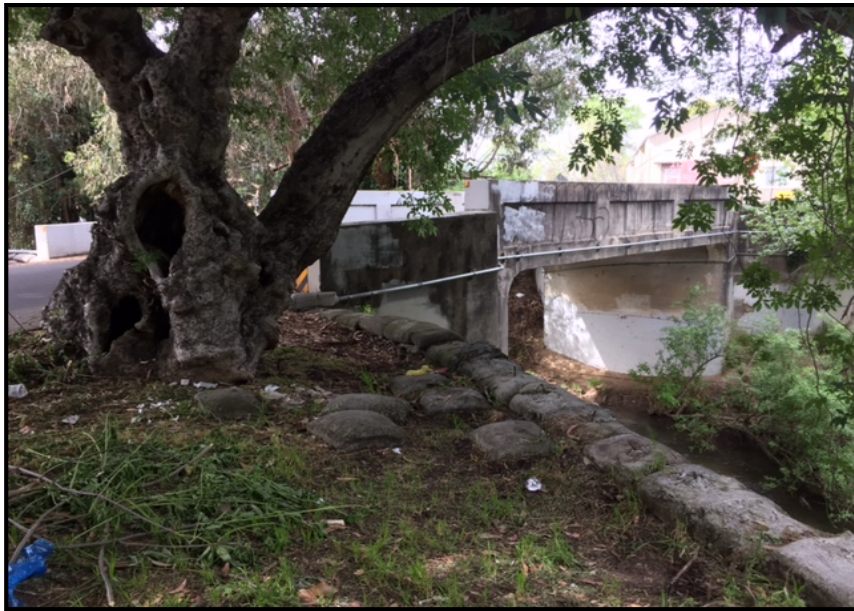
View from PA looking NE.
