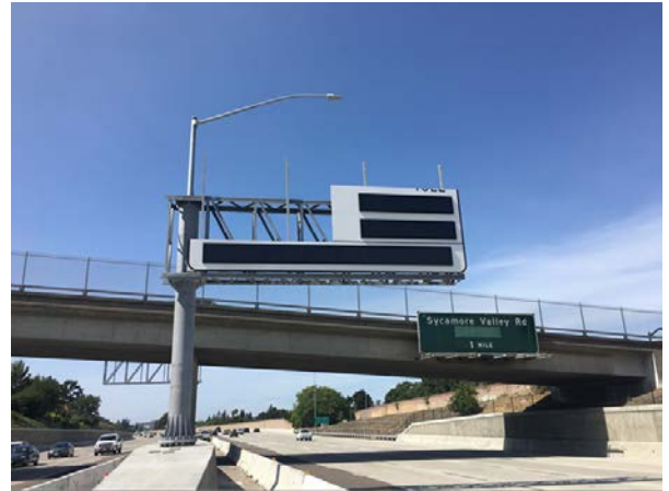
A newly installed overhead toll sign.
