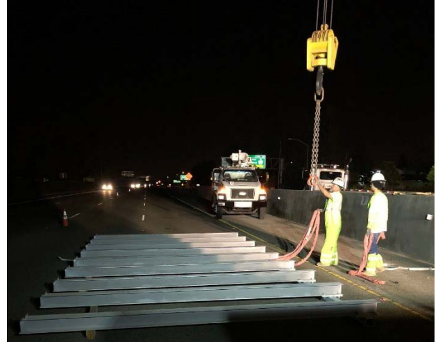
Sign structure installation
