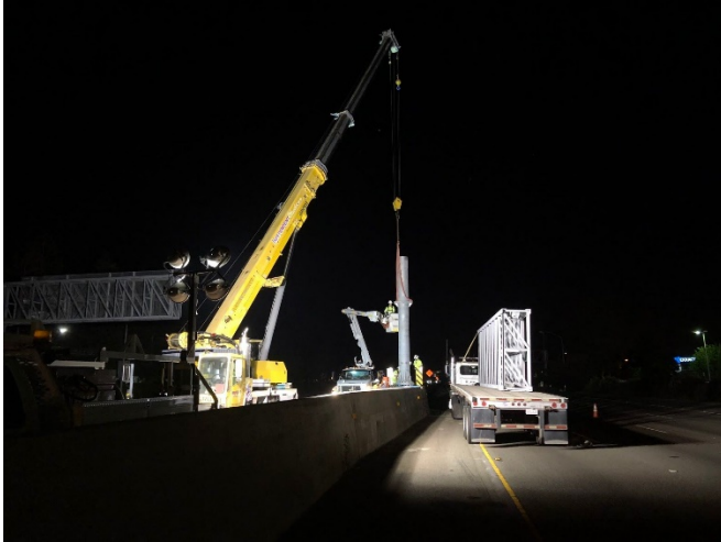
Sign Structure & Pole Placement
