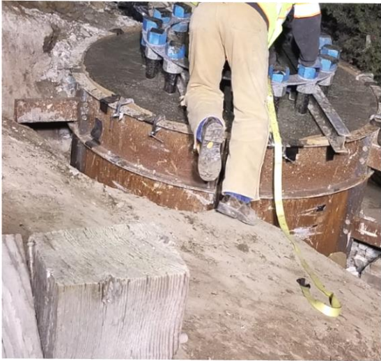
Finishing concrete on sign-bridge pedestal
