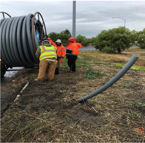
Installing Toll System Communications Equipment
