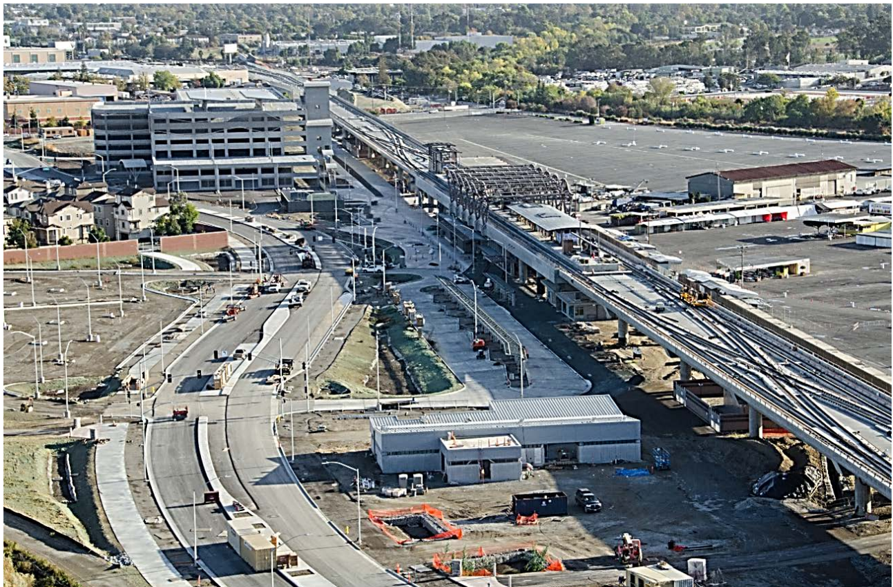
(VTA: BART to Warm Springs, Berryessa Extension)
