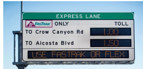
VTMS Displaying Tolling Information
