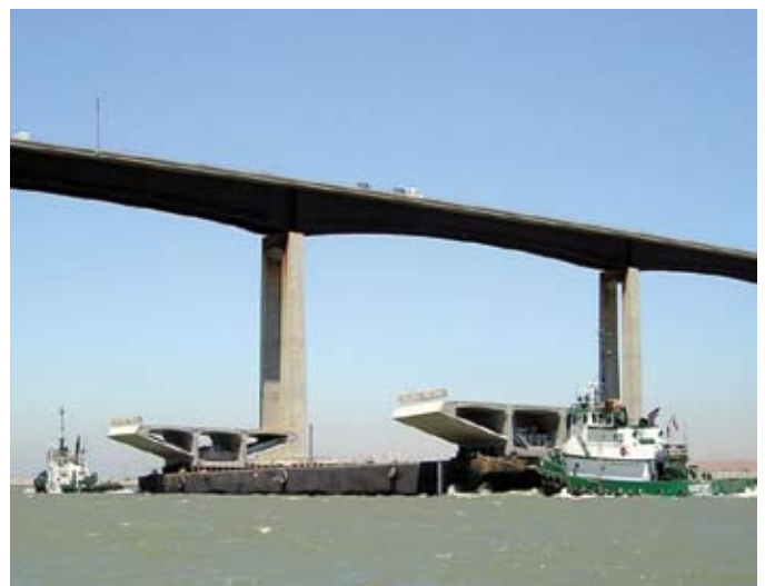
Two segments make their way to the construction site.
