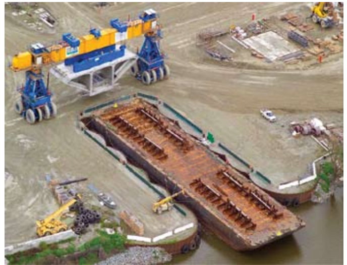
Straddle carrier loads a segment on a barge.
