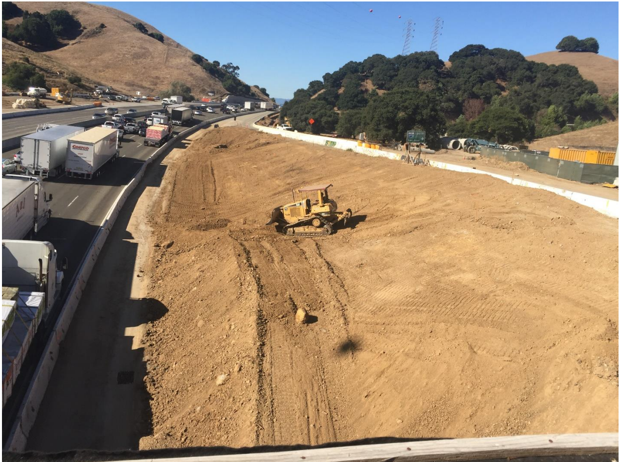
I-680 Sunol Express Lane Project (Phase 1) under construction
