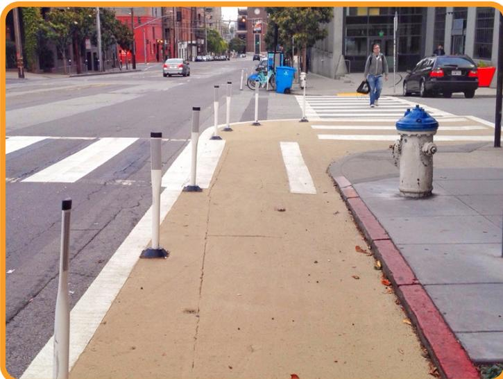
A Painted Safety Zone (PSZ) is an area around a pedestrian crossing where paint and plastic posts have been applied in the roadway. A PSZ helps to increase pedestrian visibility and reduces vehicle speeds while making turns at an intersection. In Bayview-Hunters Point, many intersection locations with perpendicular parking immediately adjacent to the crosswalk have been identified for a PSZ.
