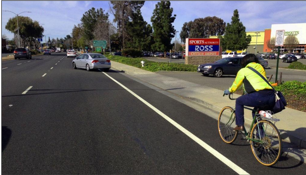
Figure 62 Bike Lanes on El Camino Real in Sunnyvale, Installed in 2015
