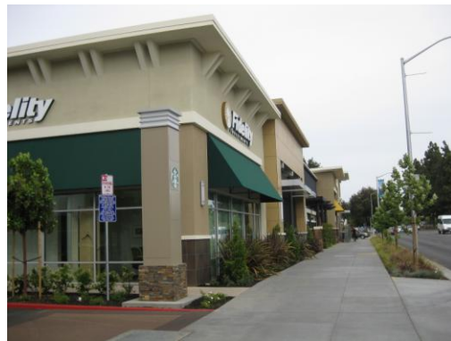
Streetscape improvements on El Camino Real, provided in Phase I of the San Antonio Center project.
