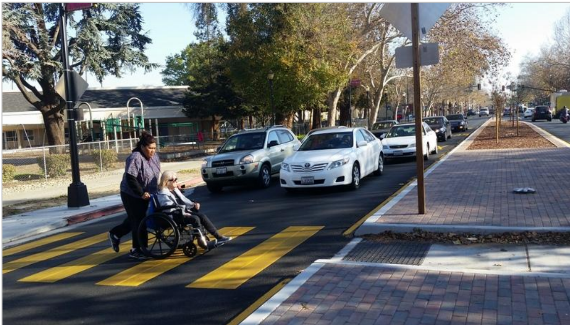
Figure 34 The Alameda features a Road Diet, Bulbouts, Landscaped Median, and Continental Crosswalks
