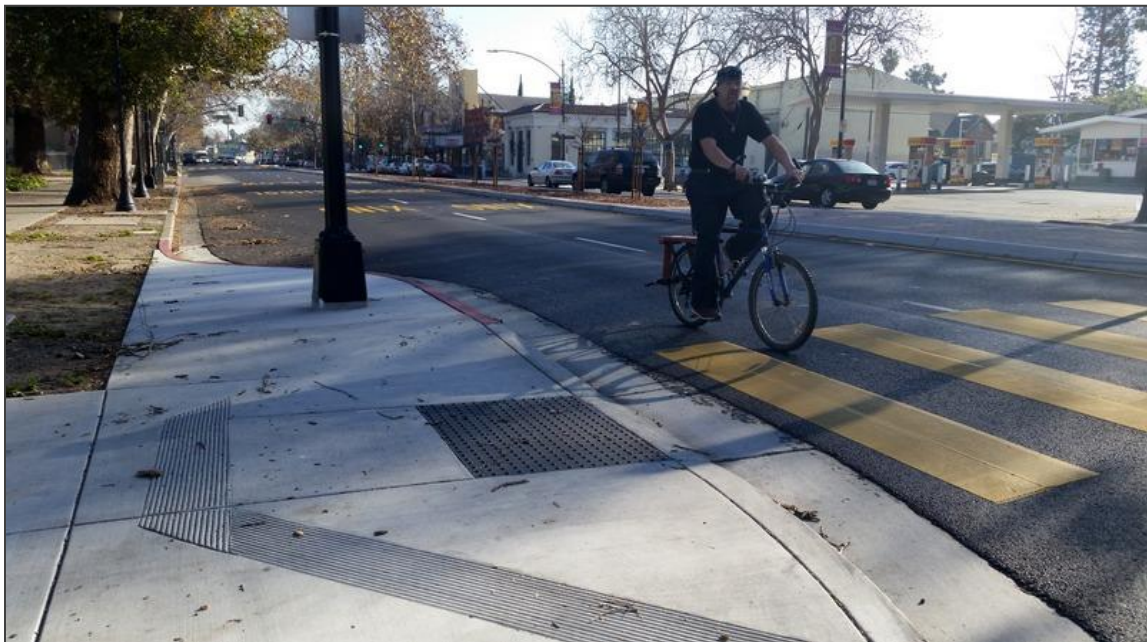
Figure 15 Relinquished Portion of The Alameda (Formerly SR 82) in San Jose After Streetscape Redesign, With Bulbouts and Wide Pedestrian Refuge Islands
