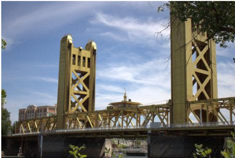
Figure 57 SR 275 / Tower Bridge
