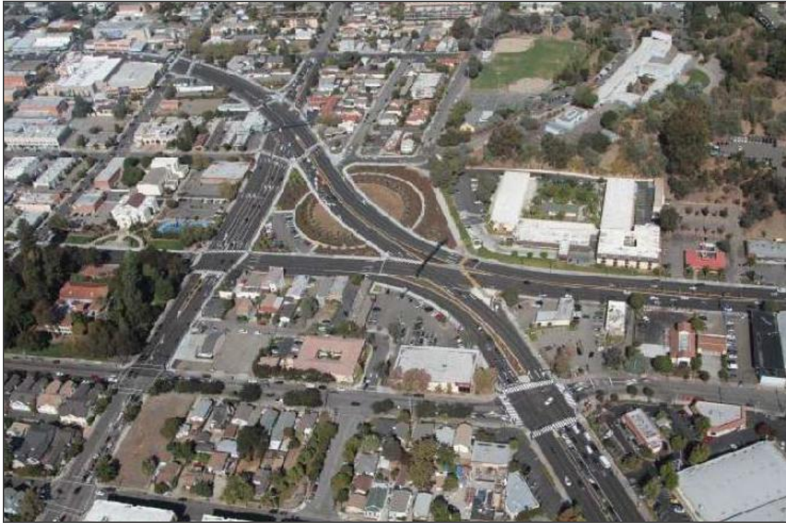
Figure 30 Aerial View of the Relinquished Roadways in Hayward
