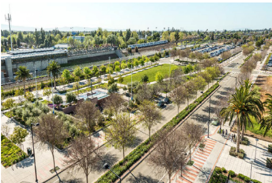
Figure ES-1: East Entrance to the Union City BART Station
