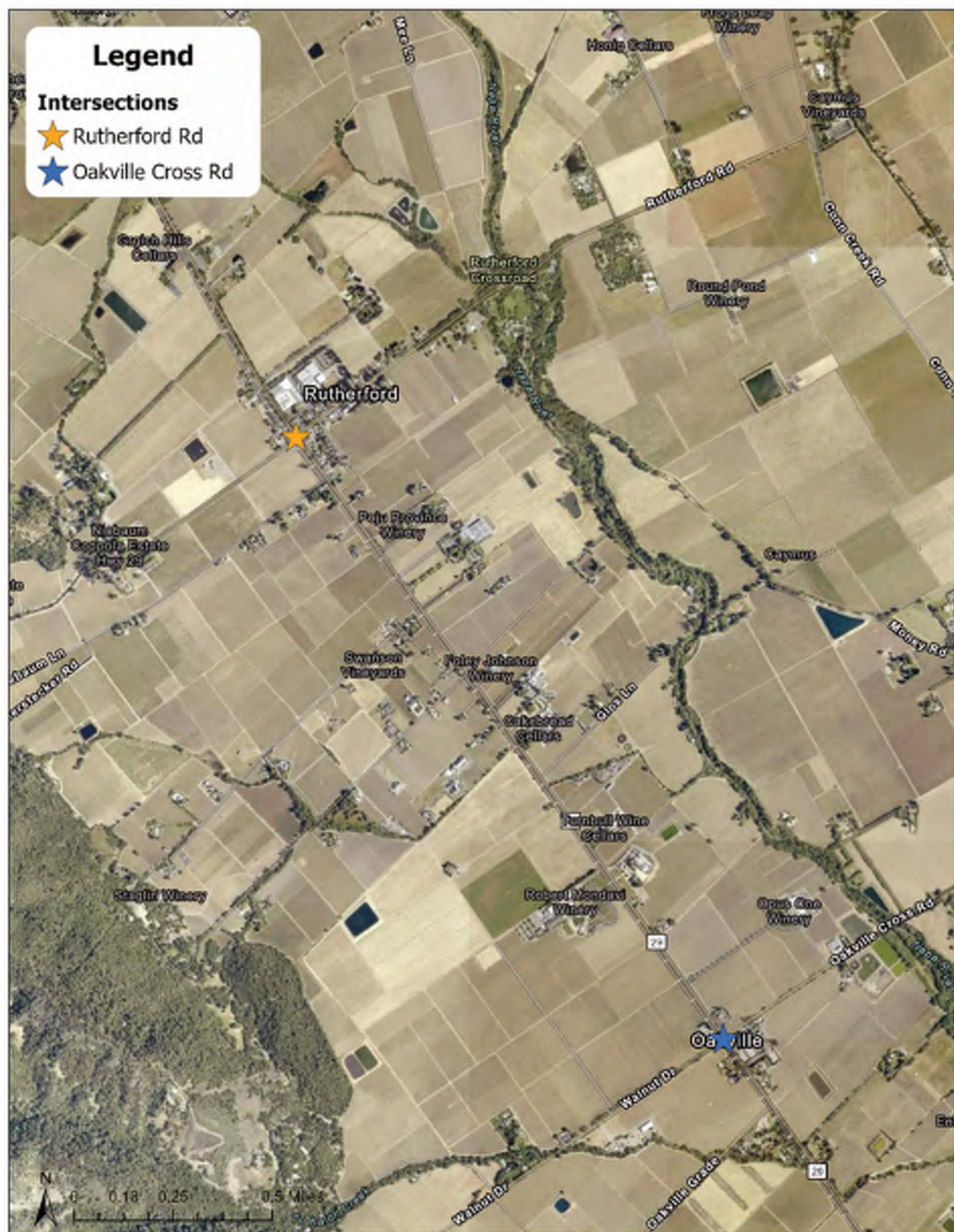
Figure 1. Aerial View of Project Location at each Intersection, 2023
