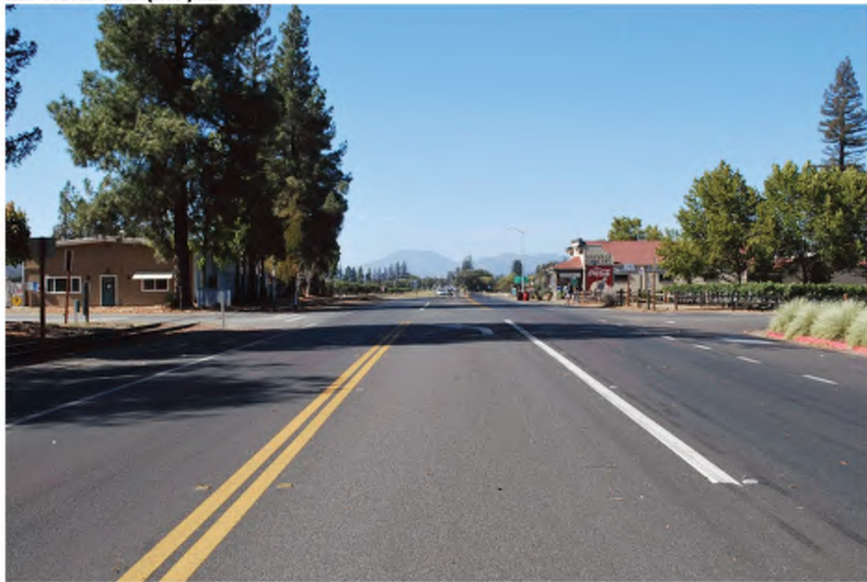
Figure 3. Looking Northwest from the Intersection at Oakville Cross Road and SR 29
