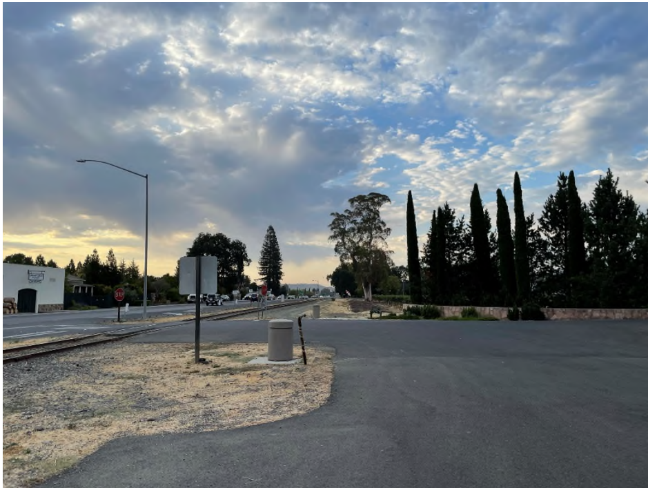
Photo 4: Project site, facing south at intersection of SR-29 and Rutherford Rd along railroad right of way.
