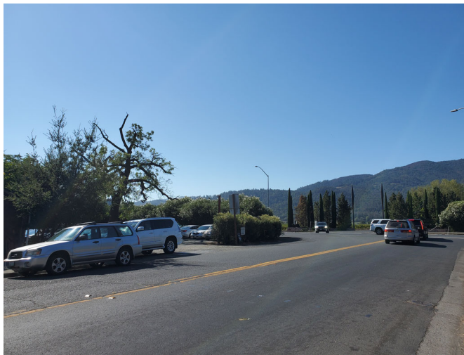
Photo 5 – Rutherford Road/SR-29 Intersection, looking southwest
