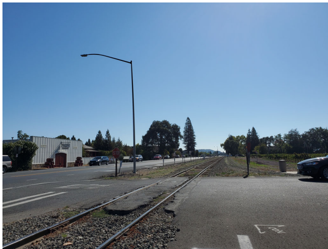
Photo 6 – Railroad along Southbound SR-29 Opposite Rutherford Road, looking south
