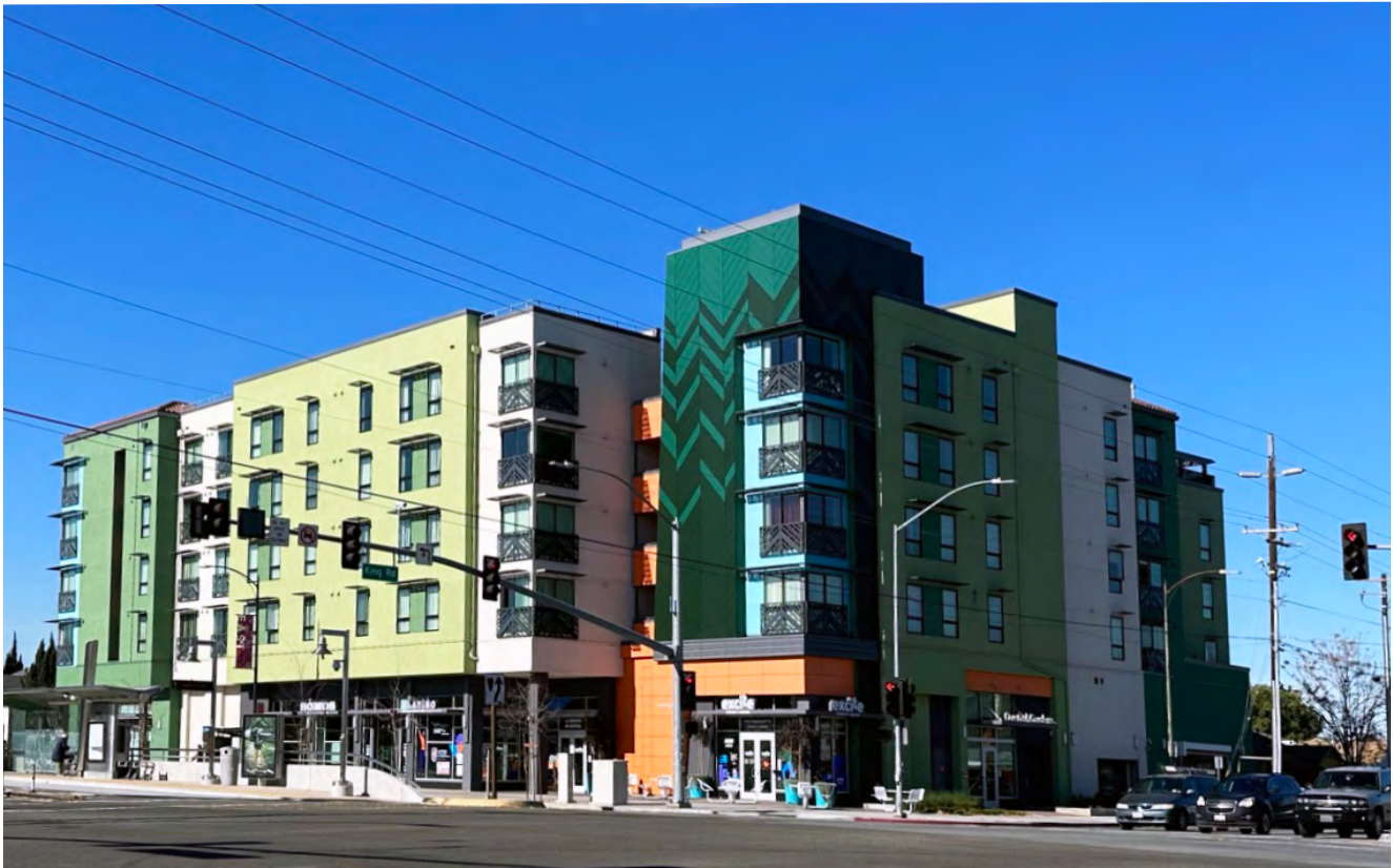
Affordable housing apartment building, Santa Clara County Photo: Courtesy of Resources for Community Development
