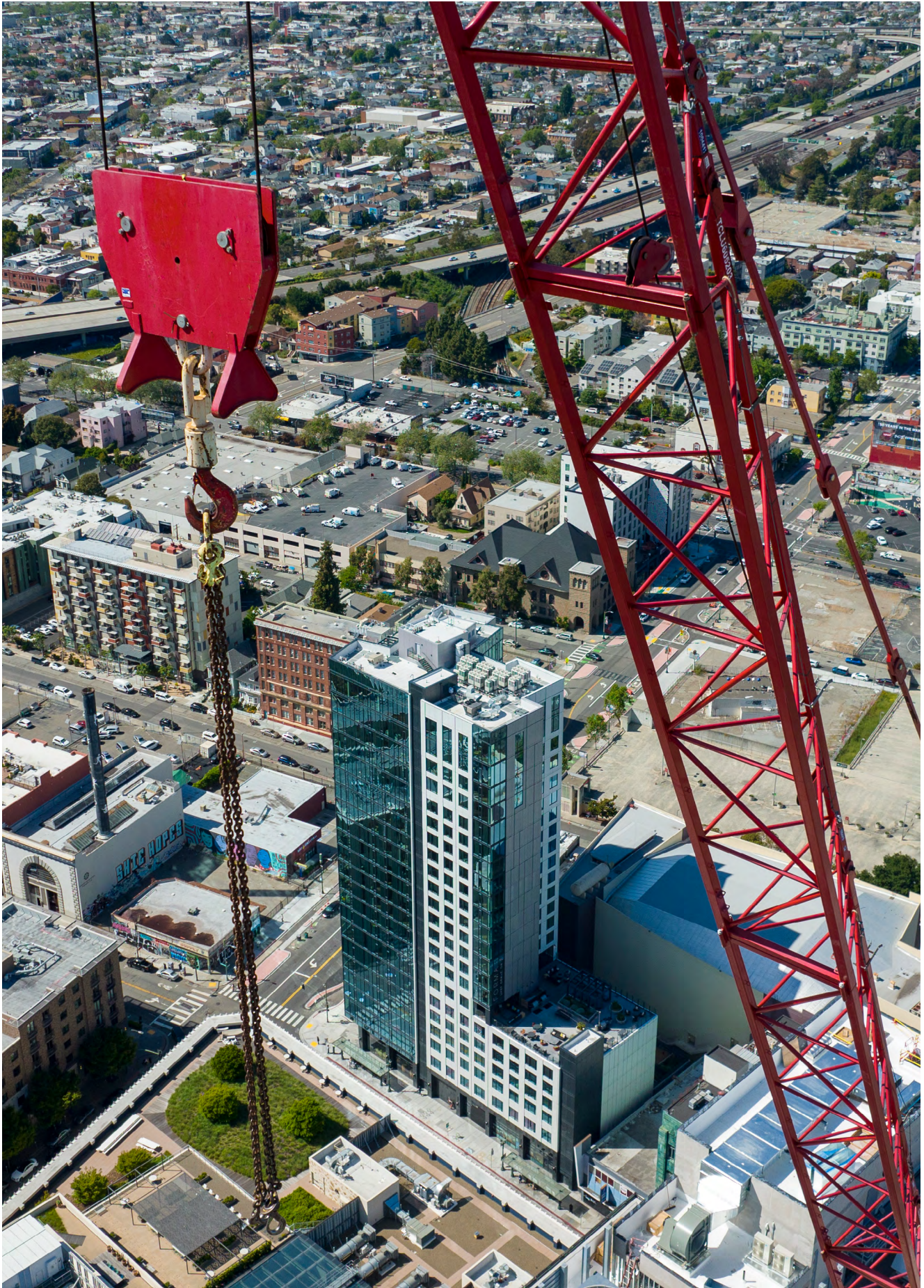
High-rise apartment, Oakland Photo: Karl Nielsen
