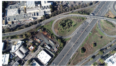
101/San Antonio Interchange – Lack of SB On-Ramp
