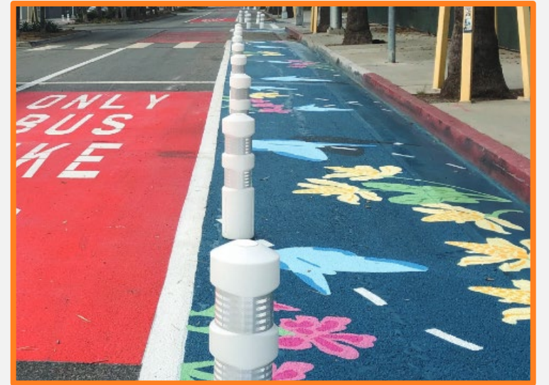
Painted transit lane, bollards
