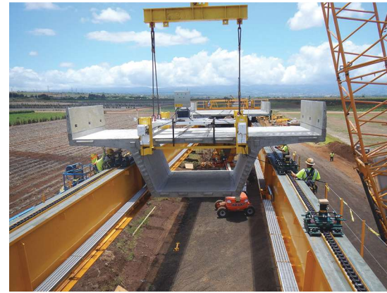
Precast concrete segments, 30 ft wide and weighing 36 tons, were cast in a facility that was approximately 5 miles away, then delivered to the site for erection on underslung girders.
