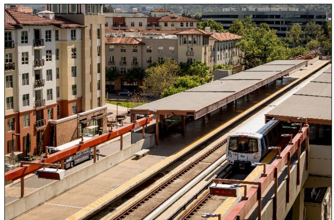
Contra Costa Centre Priority Development Area
